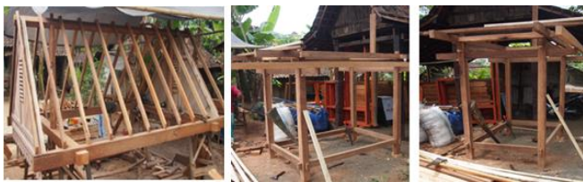
Figure 4. Roof and Prop Component from House of Using
