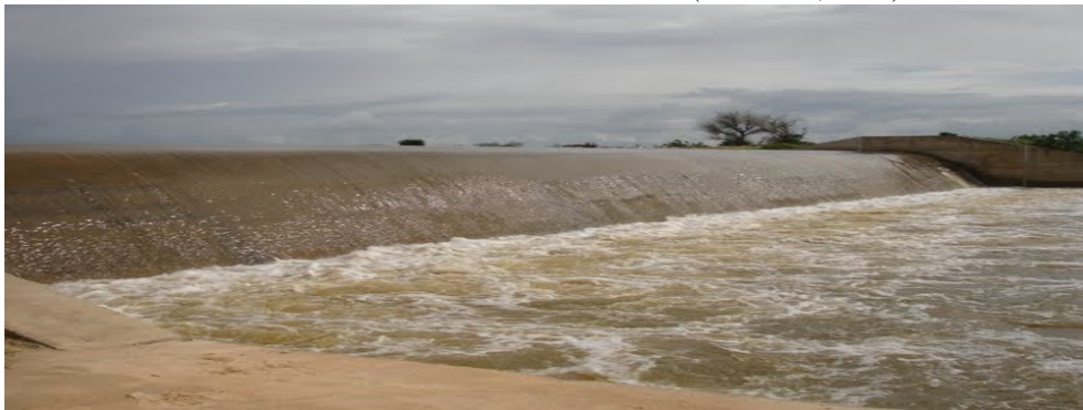
PLATE 2: ALAU DAM OVER FLOW CHAMBER (SURVEY, 2013)
