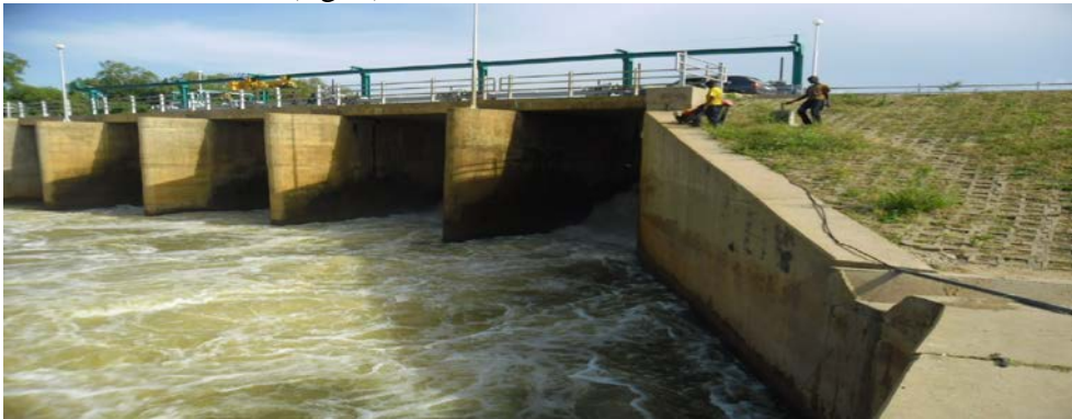
PLATE 1: ALAU DAM FLOOD GATES (SURVEY, 2013)
