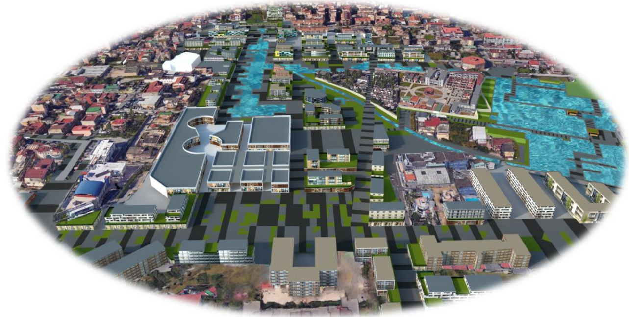
Figure 3: WSUD approach implemented in an Urban renewal case study: surface disposal network in heavy rain conditions. Source: Carbone, Corrado, De Nicola and Faiella, 2017.
