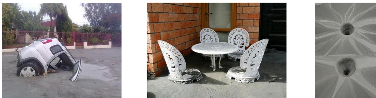
**Figure 5:** Sinking of a car and chairs for loss of bearing capacity and sand boils produced by soil liquefaction
