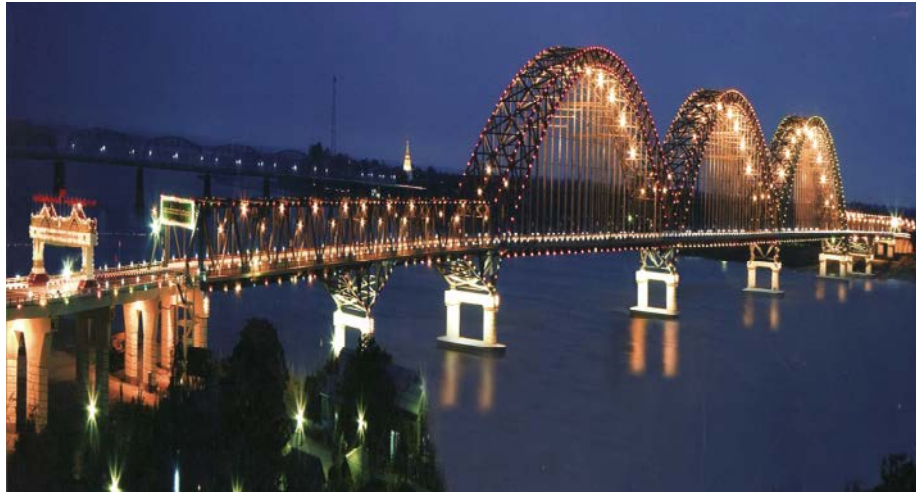
Figure 2: Ayeyarwady Bridge (Yadanarbon)
