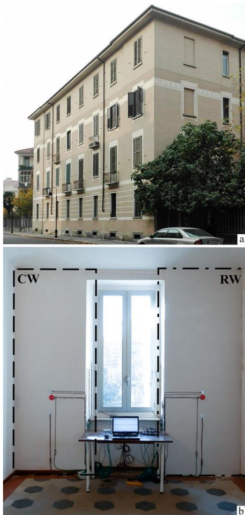
Figure 1: a) the demonstration building; b) the two monitored wall configurations;
