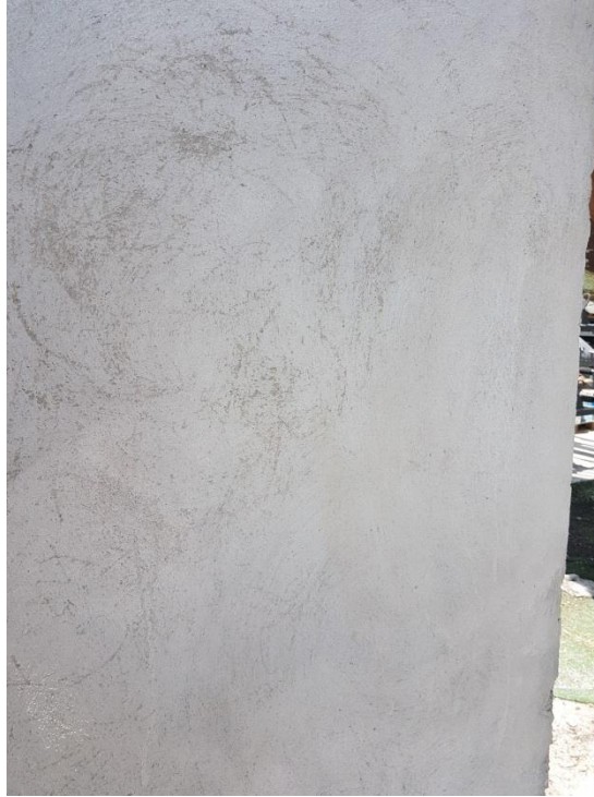
Figure 127: Pouring plaster results after two days from its application on panel.
