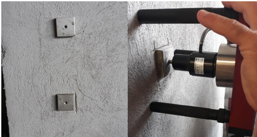
Figure 132: Left: Test plate mounted onto plaster; Right: Pull out test conducted.
