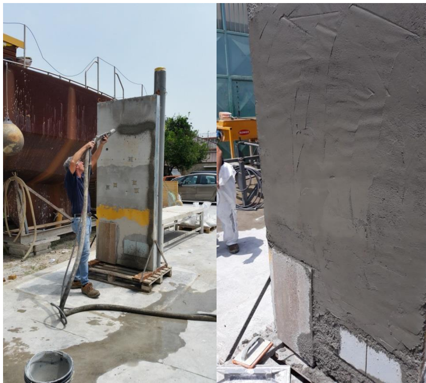
Figure 126: Left: Plaster pouring on vertical panel. Right: final results after pouring.
