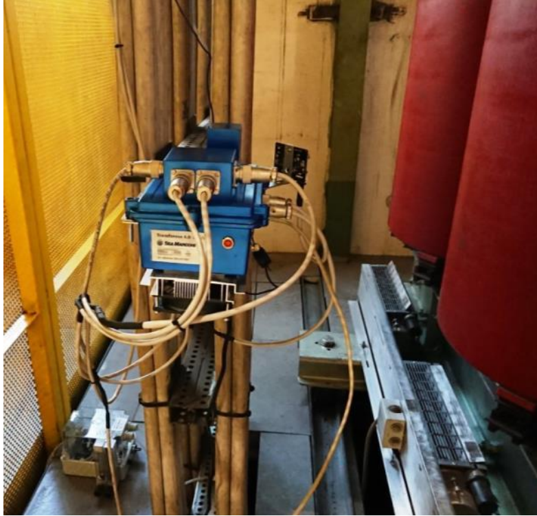
Figure 8. Installation of one of the second prototype (slave module)
