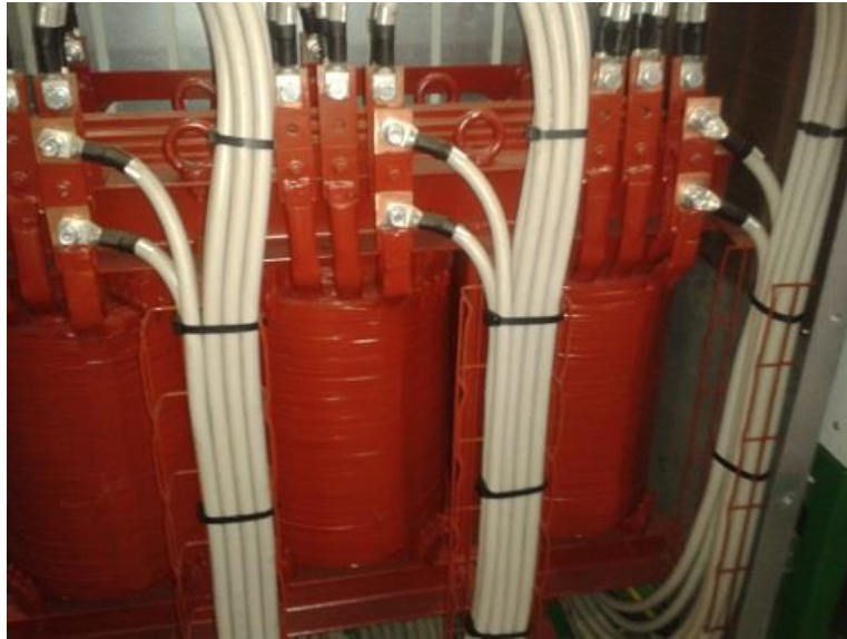
Figure 5. Example of a cast resin transformer (250 kVA)
