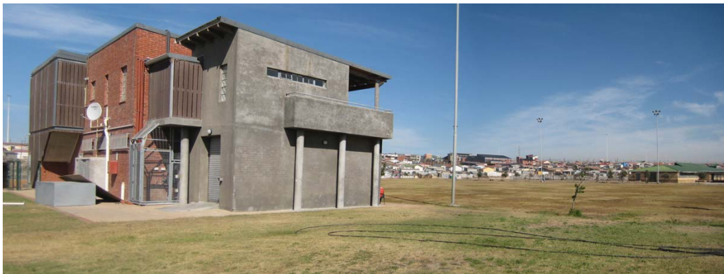
Fig. 138: Kwamfundo sport facility, 2017 545
