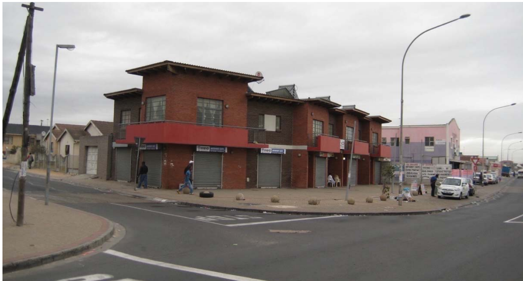
Fig. 123: Station live-work units, 2017 530
