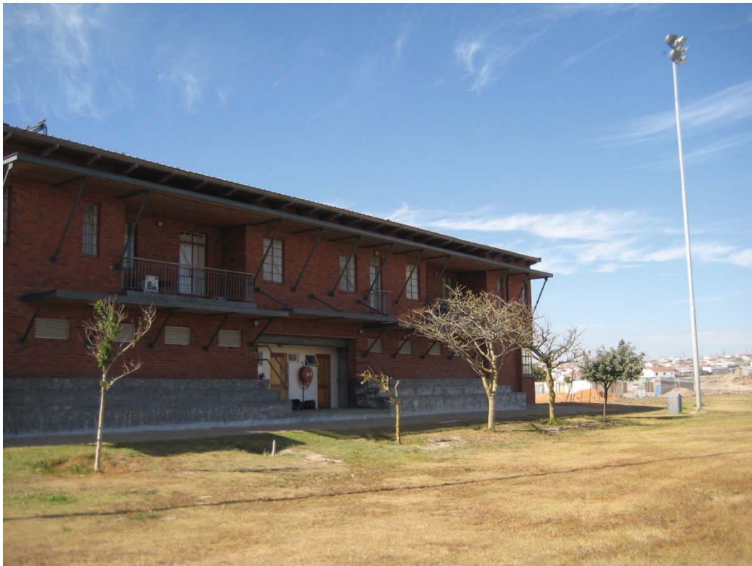
Fig. 137: Kwamfundo sport facility, 2017 544
