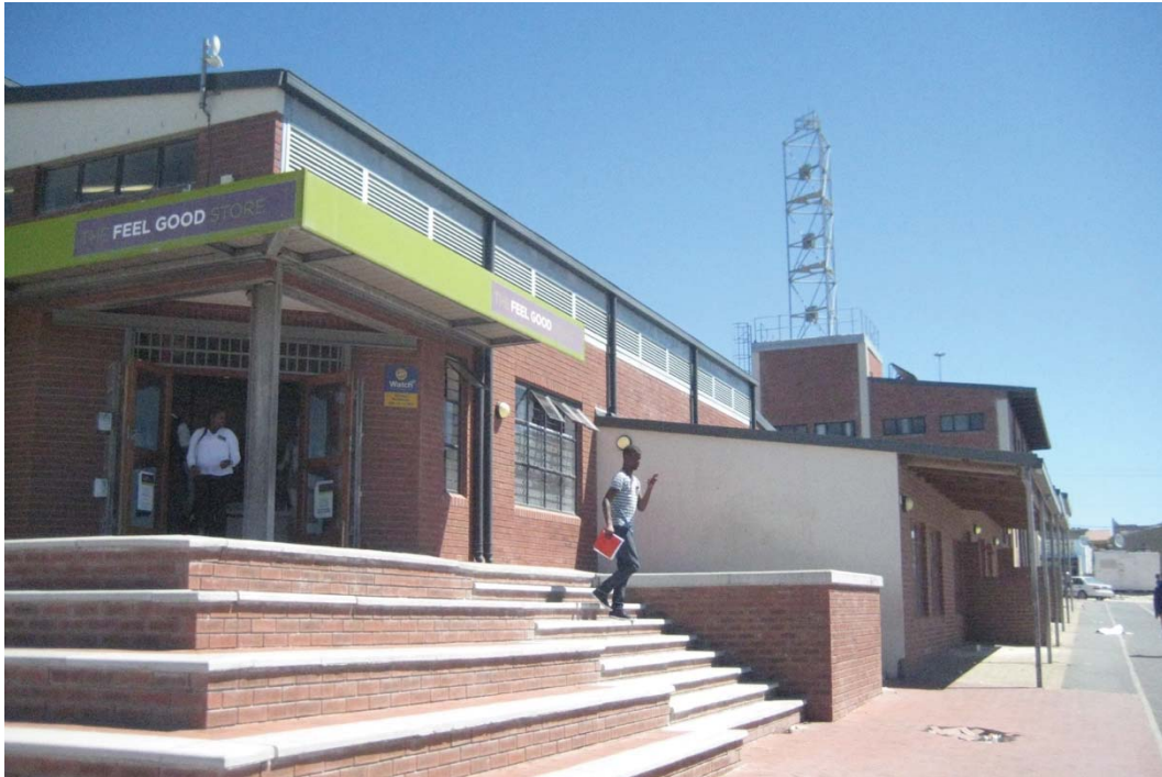
Fig. 143: Another side of the business hub, 2017 550
