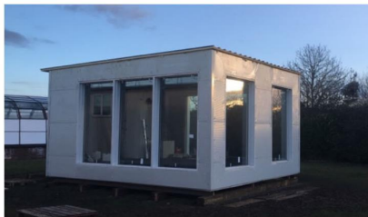
► Fig. 1: View of the west side of MATELab
