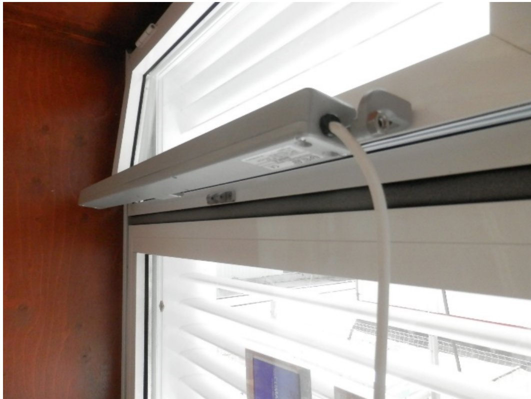
Figure 1 - Automated openings integrated in a façade element. Source: CommONEnergy project
