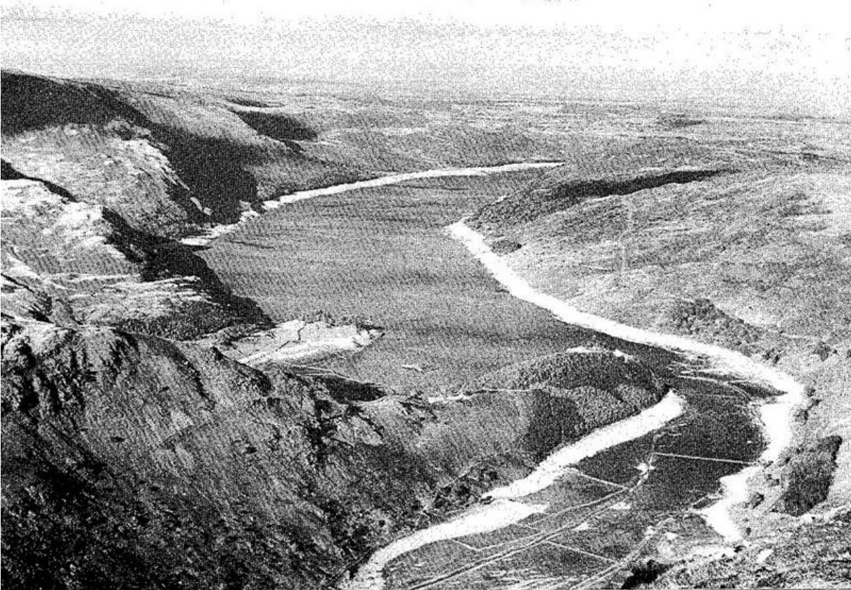
Rim effect, caused by the changing water level in a similar reservoir
