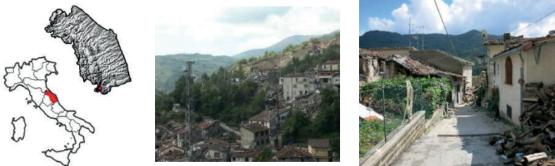
Figure 3. Pescara del Tronto in Arquata del Tronto municipality (Ascoli Piceno), is one of the perched villages allocated across the Apennines mountain in Marche region (left, center), center Italy, on the border with regions Abruzzo, Lazio, Umbria. It was destroyed by the reiterated seismic shocks from
