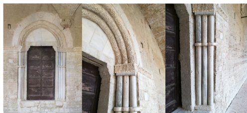
Figure 2. The portal in the cloister of the Duomo Vecchio
