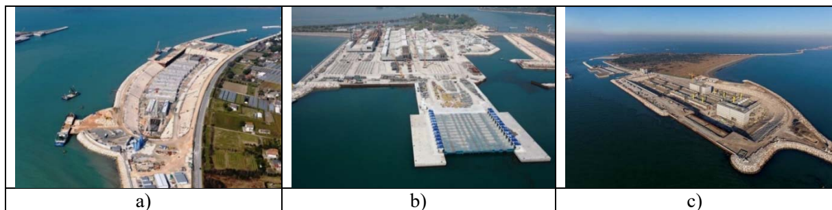
Figure 3. Precast yards. (a) Lido Treporti; (b) Malamocco embankment; (c) Chioggia.
