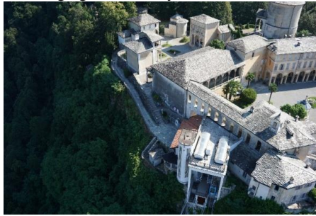
Figure 3. Oblique image taken with UAV. Western walls not detectable with LiDAR.
