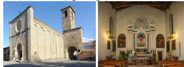
Figure 2. External (left) and internal (right) view of S. Agostino before the earthquakes
