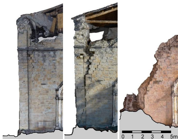
Figure 14. Orthoimages of the main façade in t1, t2, t3.
