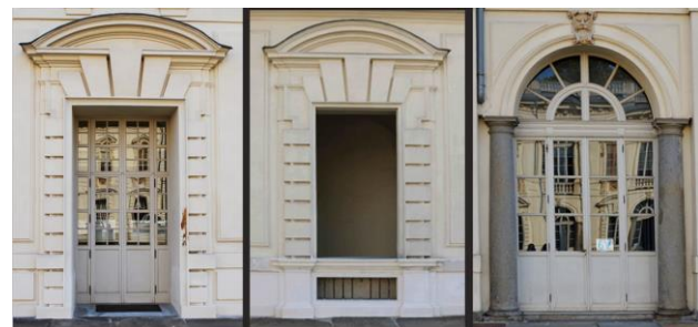
Figure 2. View of some of the analyzed architectural elements
