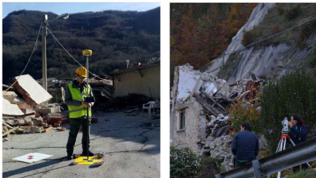
Figure 2. Survey operation with the Geomax Zenit 35 GNSS (left), Leica TS06 total station survey (right)
