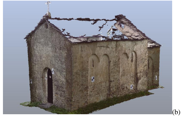
Figure 8. Original TLS point cloud (a), cleaned TLS point cloud of the Chapel (b)
