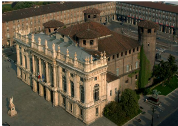
Figure 3.2: Palazzo Madama, aerial view
