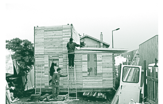
Low-cost house from scrap timber © Bois & Cie
