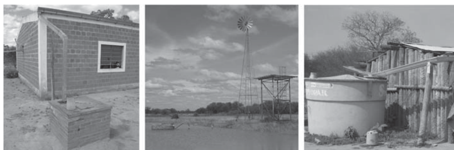
Figure 4.12: Paraguayan Chaco, April 2014. Aljibe (left), tjamar (centre) and tanque (right) (photo by E. Ponte).
