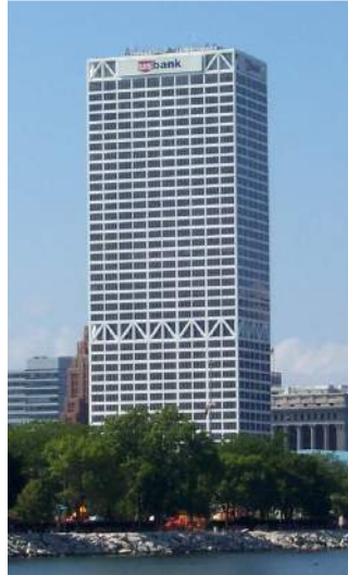
Figure 1.10 – The U.S. Bank Centre in Milwaukee (1973, USA): example of a tall building restrained by two outrigger systems.
