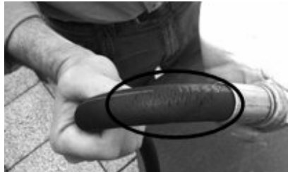
the poor condition of the broken hose
