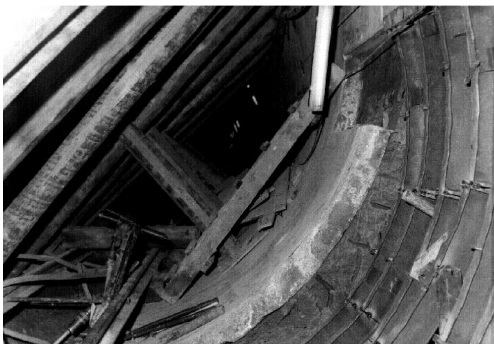
SARMENTO TUNNEL (SINNI, ITALY), 1997
