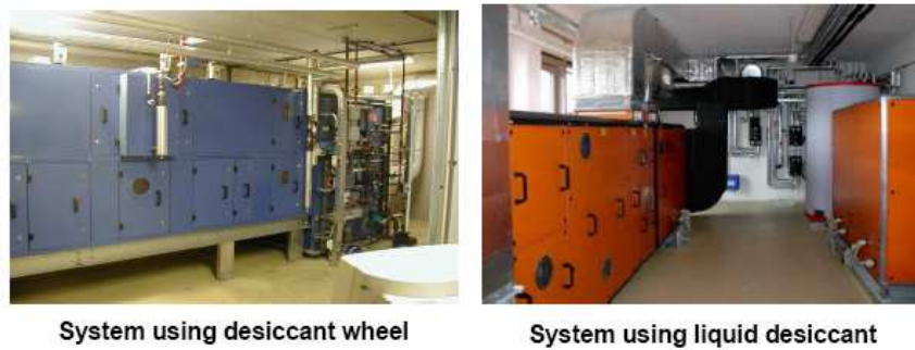
Figure 60 Open cycles-desiccant air handling units
