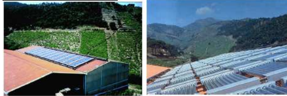
Figure 11 Wine store cooling in Banyuls, France
