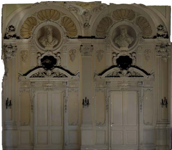
Fig. 8 – The true orthophoto of the Southern wall.
