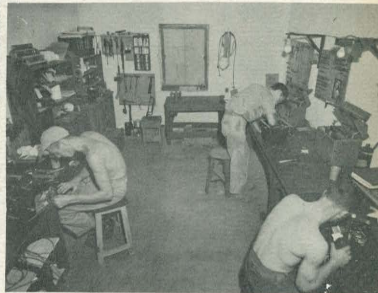
were able to catch up on much repair work . . .
