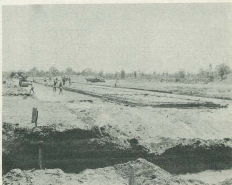
building the new taxiway . . .
