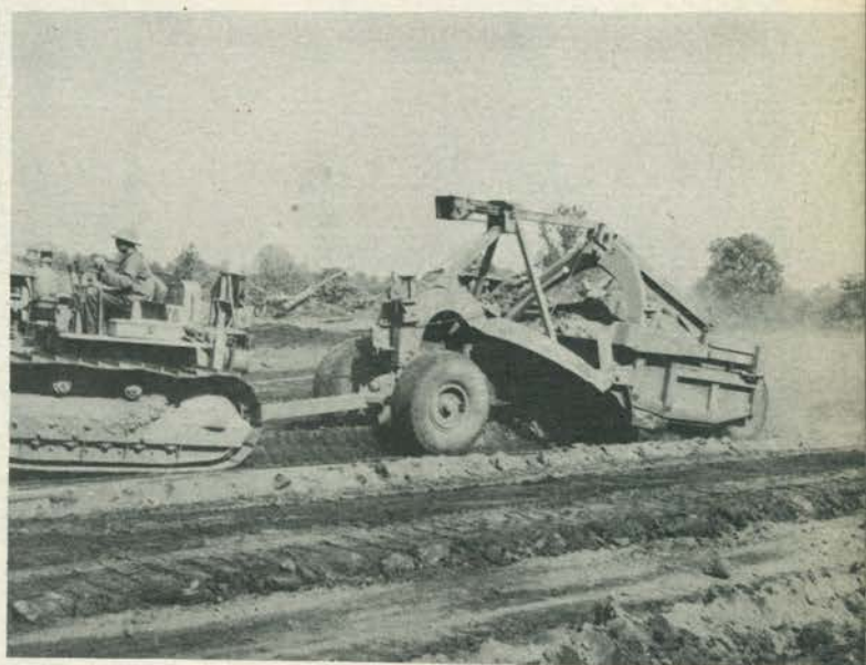
while construction work . . .
