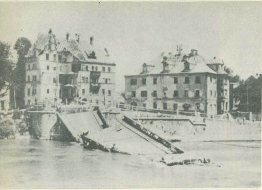
Bridges destroyed by the Germans at Regensburg
