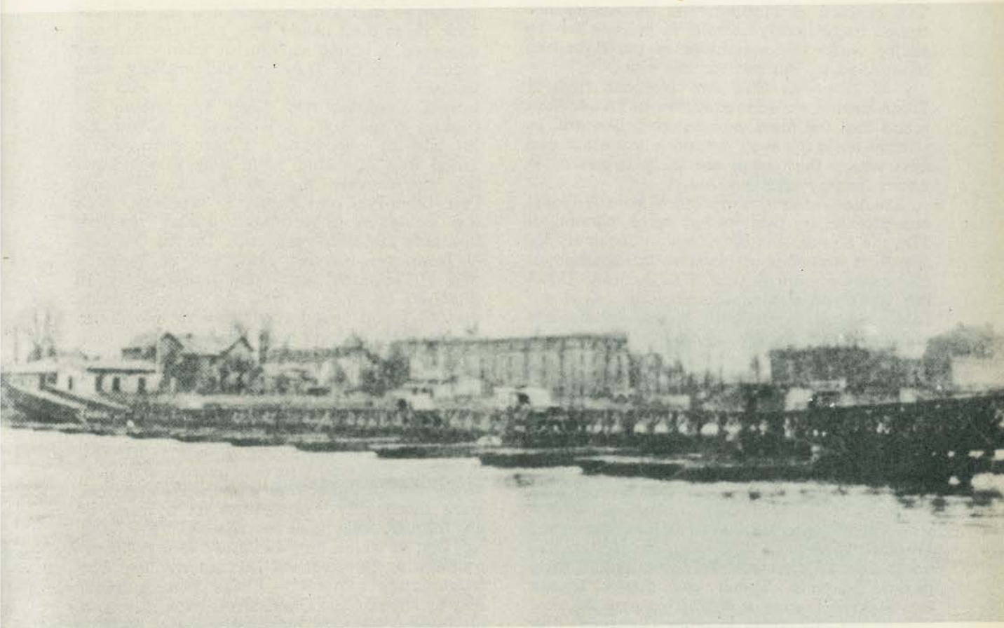
Floating Bailey Bridge at Thionville
