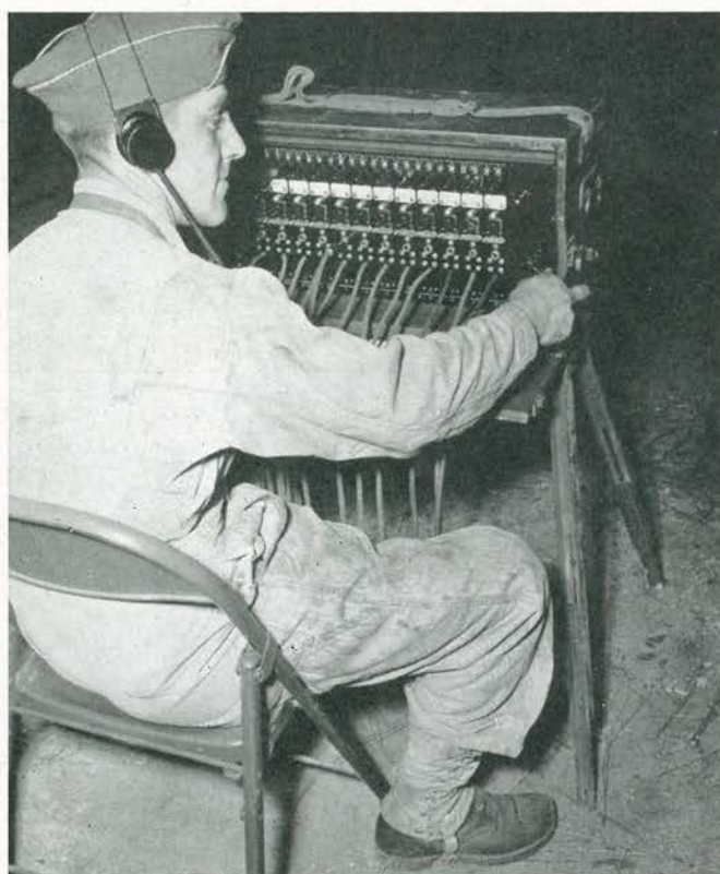
Testing lines by means of outdoor switchboard.
