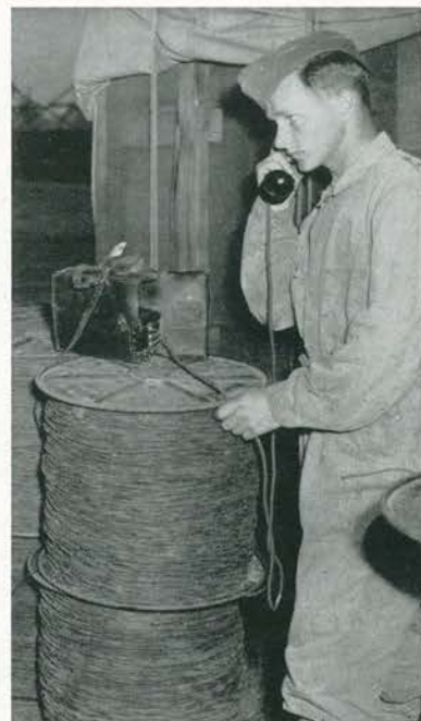
In war zones specially designed telephones are used.
