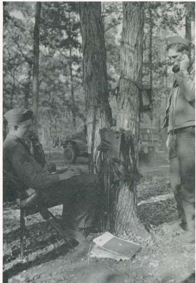
Switchboard in the field.
