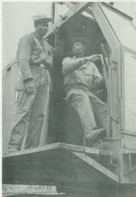
Pfc. George Mix, a slinger, looks on as Pfc. Nathan McMichael, crane operator, instructs him the operation
