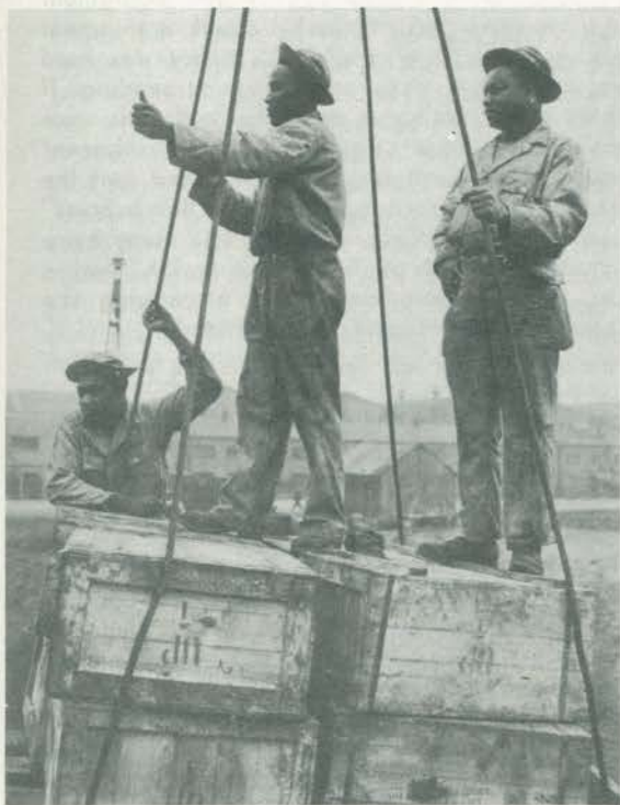
Sgt. Leslie Barns rides along side a draft of smoke bombs being hoisted by a giant crane. Pfc. J. B. Randall, a slinger, signals to the crane operator, Cpl. Vance Dunk.
