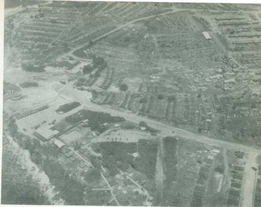
Aerial view, Base M.
