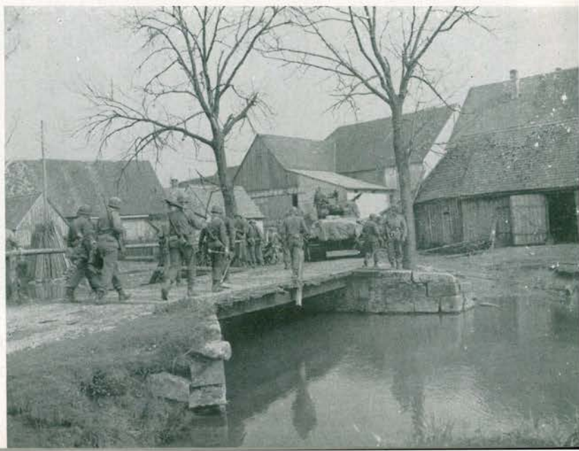
South of Neustadt on road to Nurnberg, armored infantrymen cross small bridge on stream while treadway bridge is repaired under fire.
