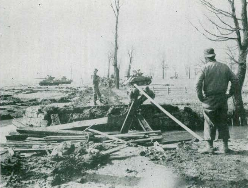
Bridging in combat—Infantry supported tank command on attack mission wait while treadway bridge is installed under fire near Dietersheim.
