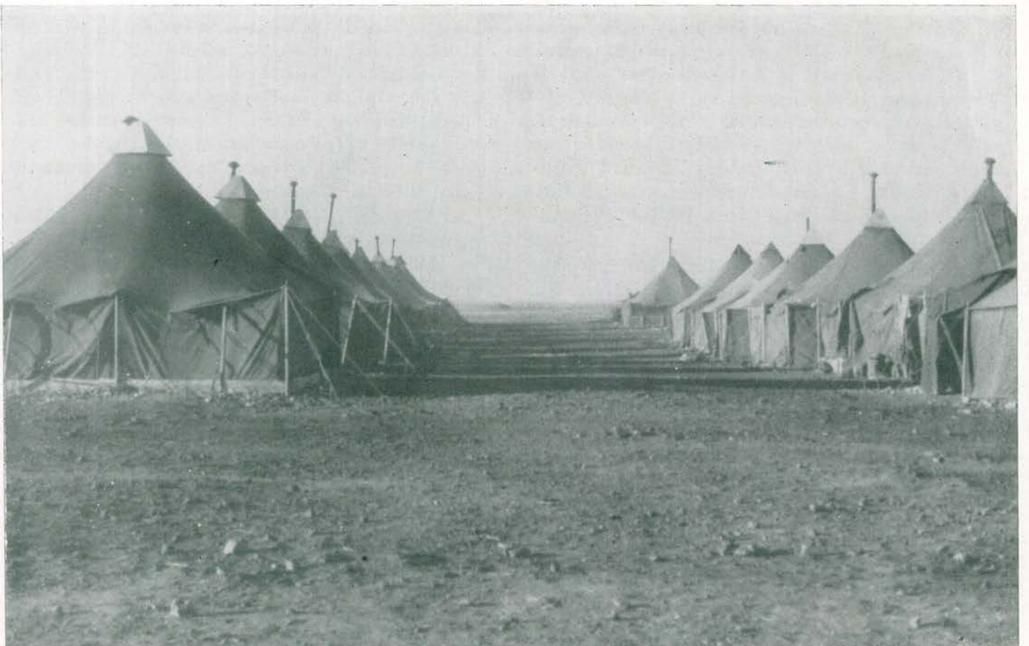
Staging Area—Marseilles, France
