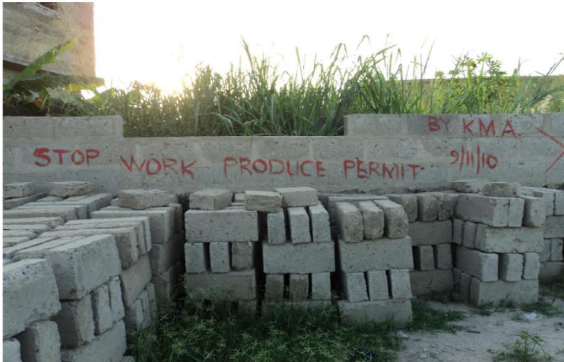
FIG. 4.3 a & b. Warning Inscription, “Stop Work Produce Permit” Or To Be Demolished Due To Flouting Of Building Regulation.
