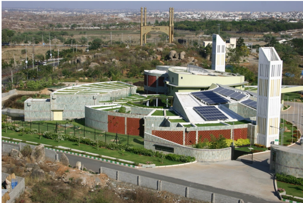
Figure-2 CII Sohrabji Godrej Green Business Centre, Hyderabad – First LEED Platinum Certified Building in India 4
