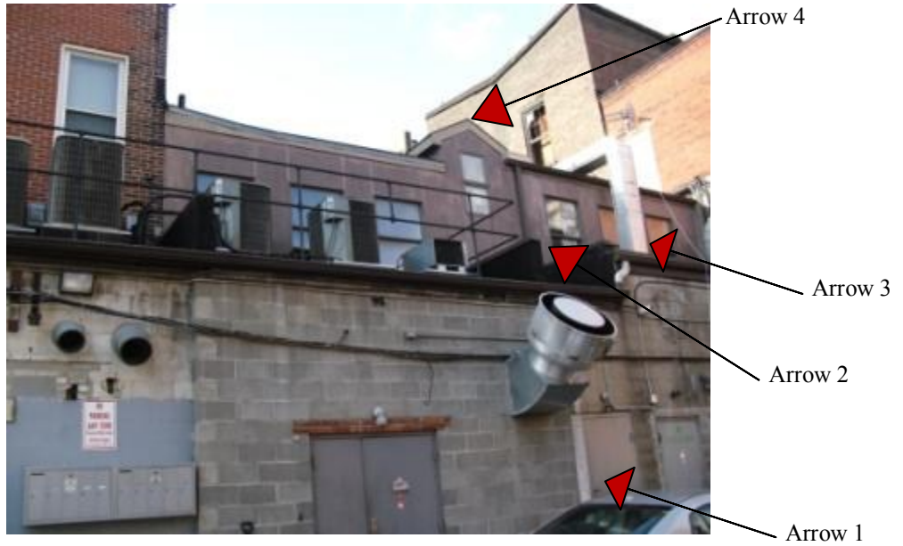
Figure 5: View of the roof from the parking lot. Access to roof was through lower door (Arrow 1), then up interior steps, through a door, into a conference room, out the window (Arrow 2), up a ladder (Arrow 3), to the control roof. The RTG is on the other side of the small peaked roof (Arrow 4). This picture illustrates why easy access to the roof is essential.
