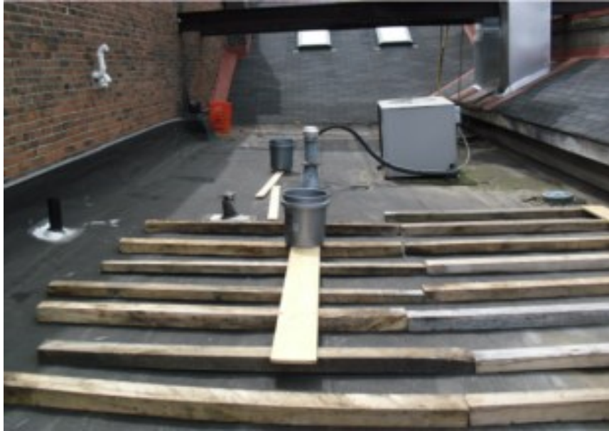
Figure 9: 4 x 4 beams as foundation.
