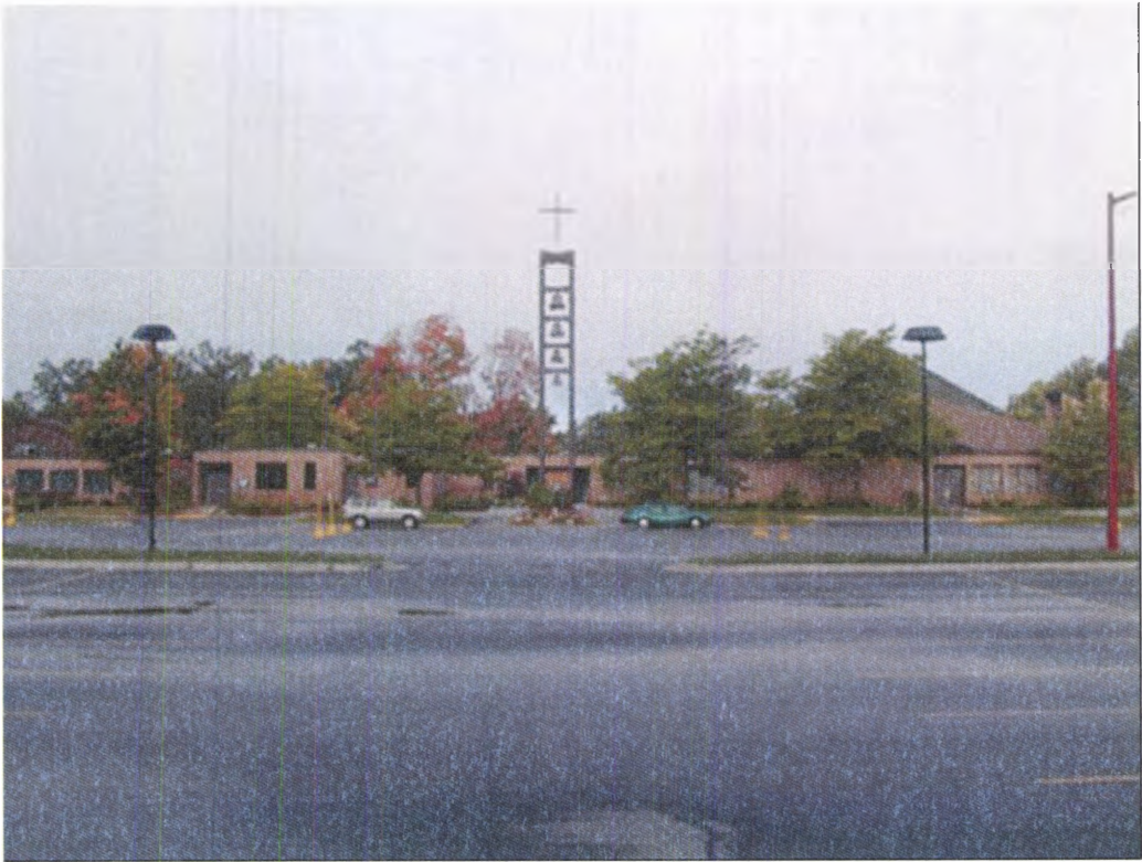
FIGURE 10: Another typical post-conciliar suburban Catholic church. Note the surrounding parking lot, and the ambiguous nature of the buildings in the background. Only the cross and bell tower distinguish this building as a Catholic church.
