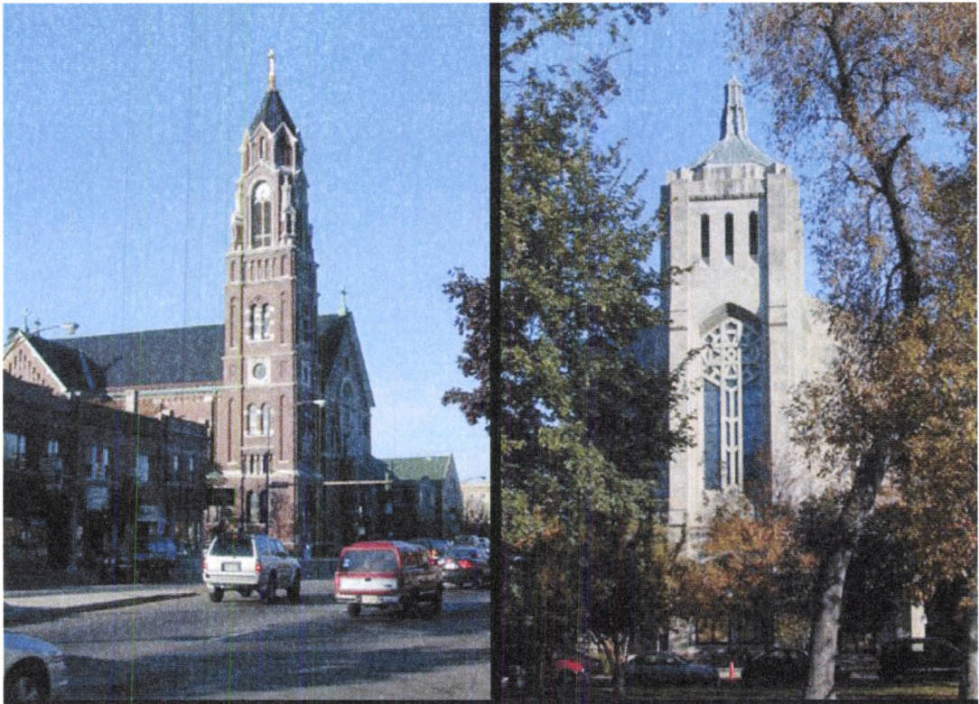
FIGURE 13: Front facades of two urban Chicago Catholic churches. St. Benedict (1909) on the left, Queen of Angels (1937) on the right. Note their close relationship to the streets in front of them, and their instant recognizability as churches.
