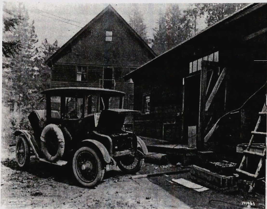
Charging the battery of a Detroit electric automobile, 1919. It was the electric cord that ultimately limited the acceptance of the electric car in America during the first two decades of the twentieth century (Library of Congress).
