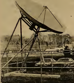
The WSMO-FM satellite receiving disc was erected on Nov. 19. The disc will be connected to the station in February.
