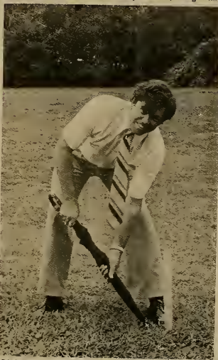
Bob Carren, associate professor of art, was the only "official" present at the groundbreaking site, Thursday, Sept. 13. He had to borrow an axe because there wasn't a shovel available. Monday bulldozers began leveling off the site of the new Arts Complex.
