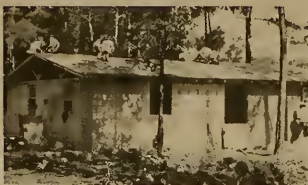
The crew rebuilding the room.
