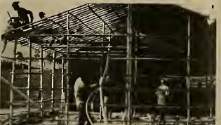
Adding a new wing to the hospital. Photo by Peggy King
