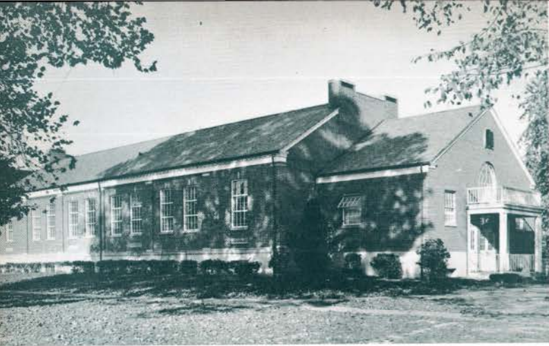
The Cafeteria and Greenhouse building was completed in 1940, making a link with Laidley and Hodges halls.
