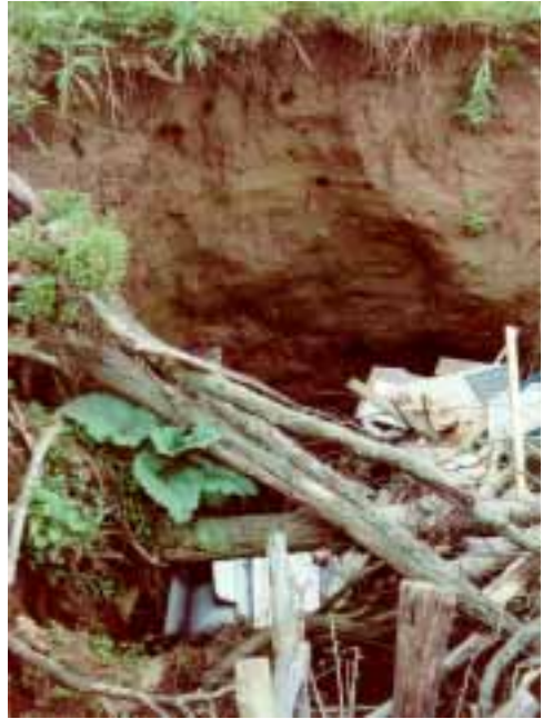
Sinkhole filled with trash and lawn debris. Photo by J.C. Currens.
