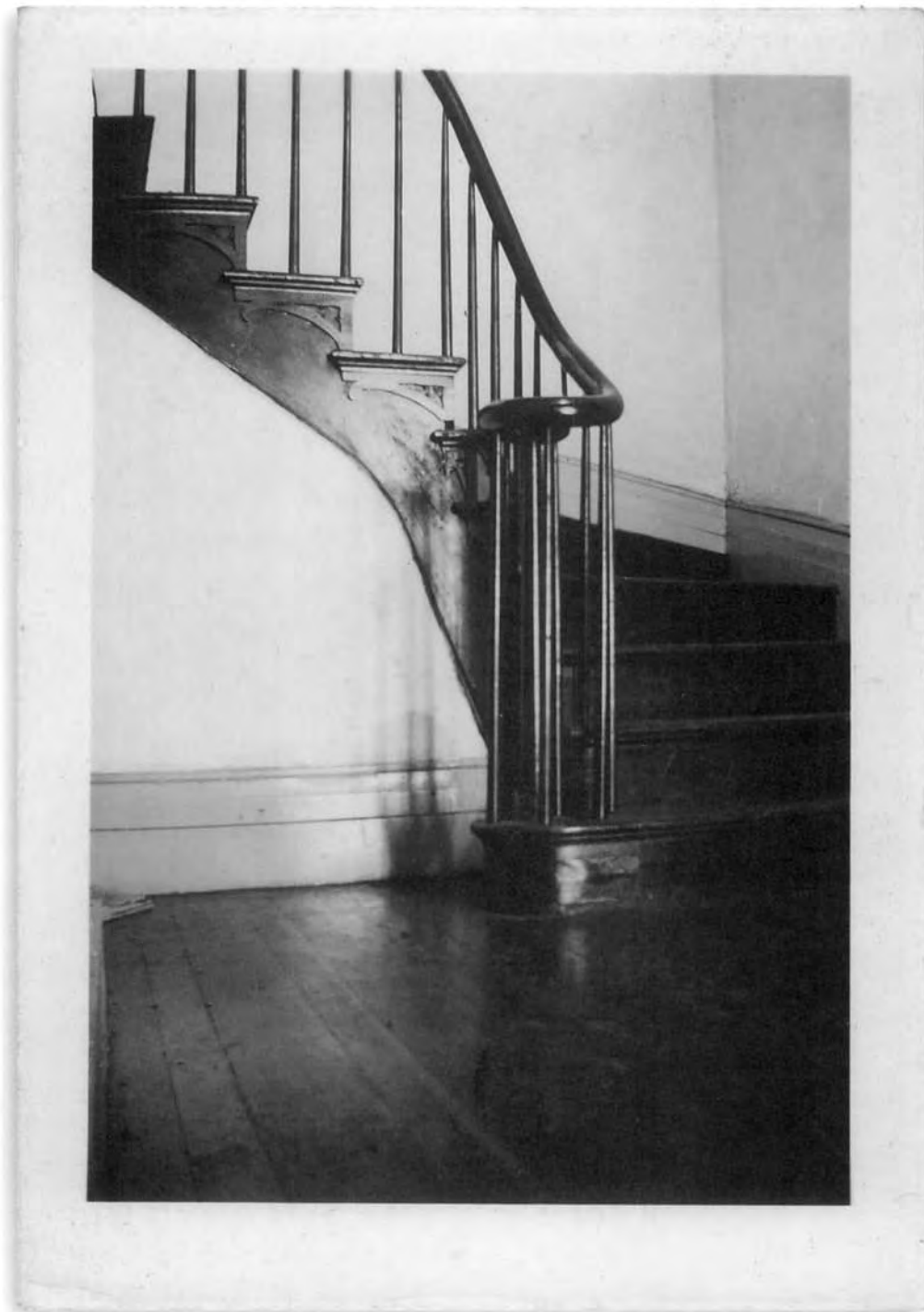
The newel for the stair at Ingelside.
