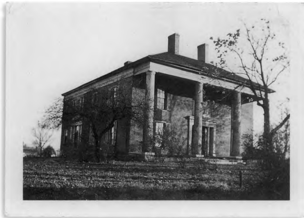
Fairview, on Nicholasville Road beyond Ash Grove Pike, was built circa 1850 for Dr. Lewis Marshall, youngest brother of Chief Justice John Marshall. It was later sold to Daniel Boone Bryan II. The masonry is Flemish bond. Fairview is one of the few Jessamine County houses with a colossal portico extending across its entire front. The house is shown in the 1940s.
