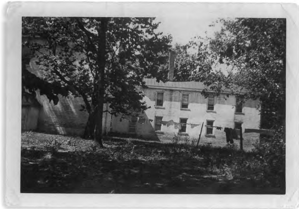
This house, in the style of architect Matthew Kennedy, stands at 312 Lancaster Avenue in Richmond. In this 1940 photograph, the original glass and leading of the doorway have been replaced with art glass of a later period. The ghost of a removed portico (probably a later addition) is plainly evident. The back section, or ell, of The Meadows, a Kennedy-style house built for Dr. Elisha Warfield in Lexington in the early 1830s, is shown. The Meadows was razed in the summer of 1960 to extend a subdivision.
