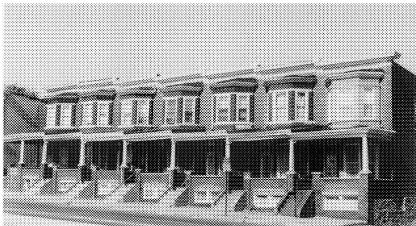
Figure 4. “Areaway” houses, among the first rowhouses on Edmondson Avenue, built in the period 1911-1914. These houses were 14 feet wide by 45 feet deep, with a narrow space (“areaway”) in the rear between every two pairs to allow light to inner rooms. (See the layout of the “areaway” style rowhouse in Figure 3.)
