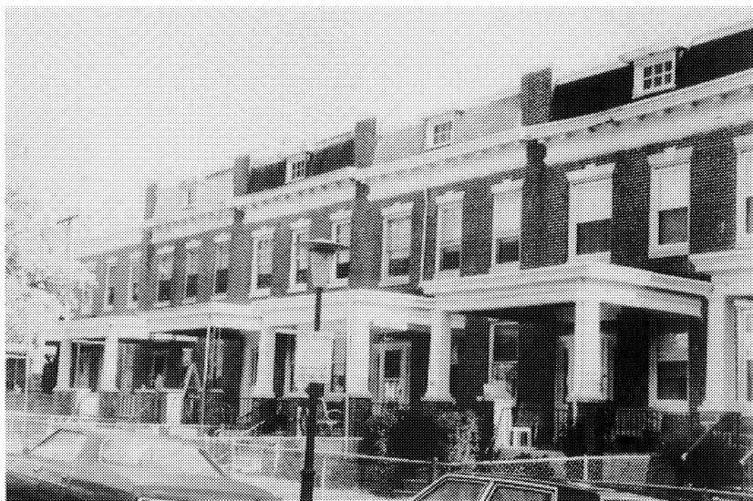
Figure 6. Daylight houses in the 500 block of Normandy Avenue built by the James Keelty Company in 1921. These were 21 feet by 35 feet. (See the Sanborn fire insurance map in figure 8 for the configuration of comparable housing on nearby N. Loudon Avenue.)
