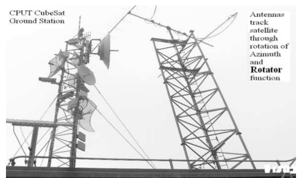
Figure 2: Antennae for satellite tracking
