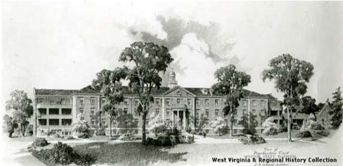
Tuberculosis building, constructed in 1940 at the left end of the lawn.
