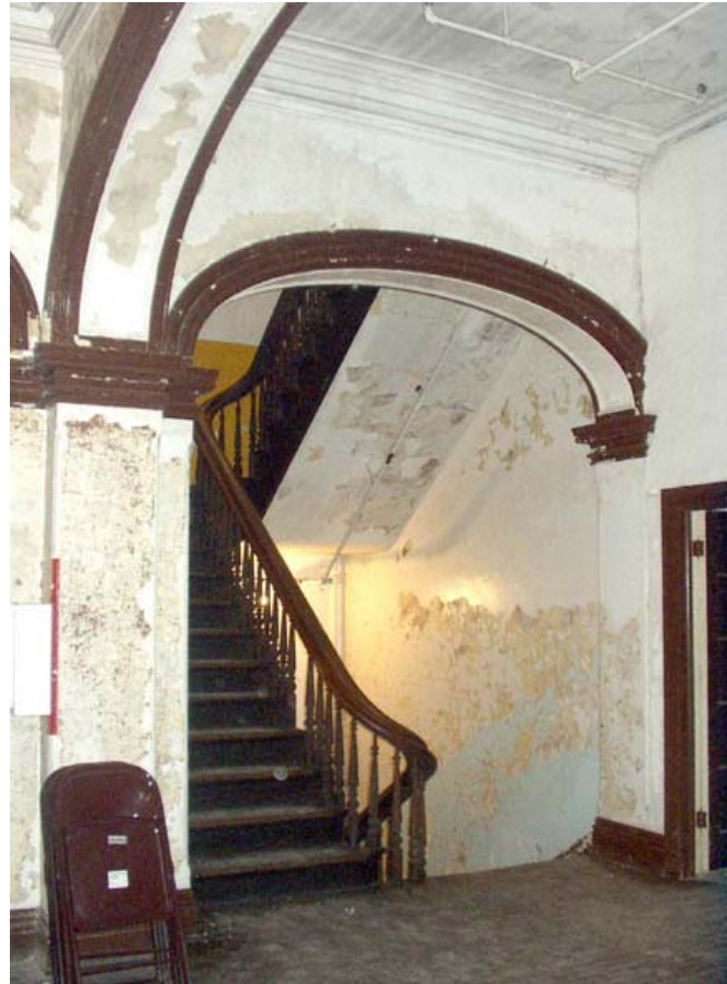
Stairway on second floor, 2008.
