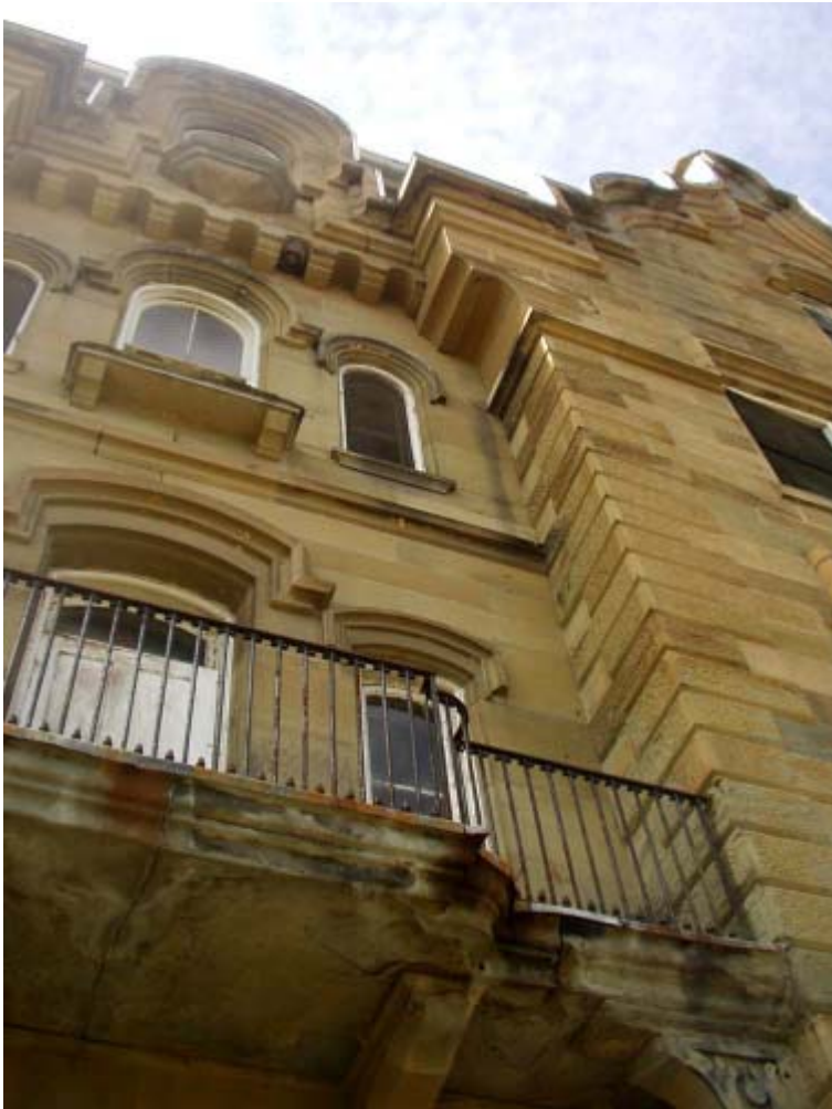
Front of the center building, viewed from porch roof, 2008.
