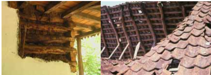
Figure 4 & 5. Construction detail of interlocking log wall and roof tiles (Source: Author)
