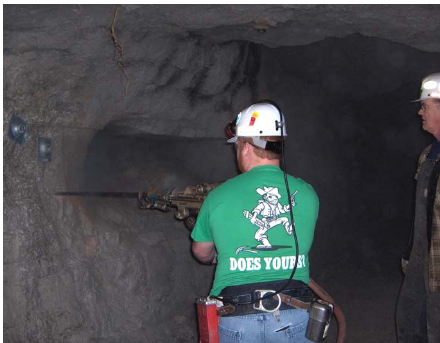
Figure 4.19. A Participant Drilling During the Underground Rockbolting Contest Under the Watchful Eye of the Missouri S&T Experimental Mine Supervisor.
