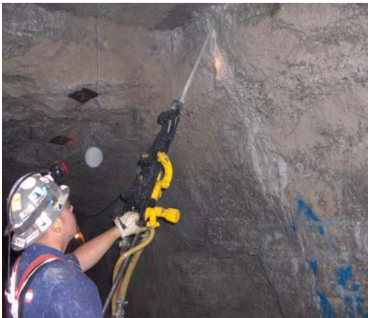
c. Drilling a Hole.
