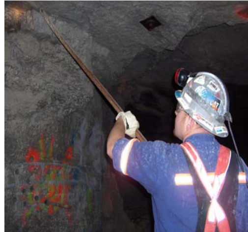
b. Scaling Loose Rock.
