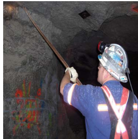
Figure 2.3. Scaling in a Mine.
