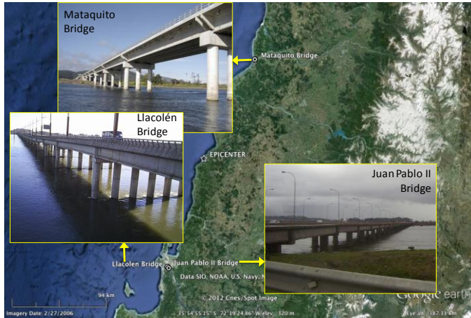
Fig. 1. Location and pre-earthquake photos of the three selected bridges.
