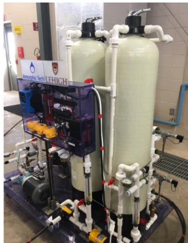
Figure 6-3. Pilot test in BNGDRF, Alamogordo, NM.
