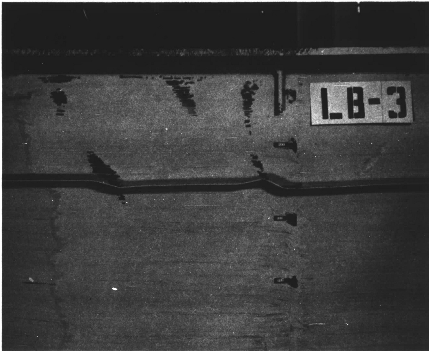
Fig. 32 Yield Pattern and Longitudinal Stiffener Buckles, Near Side (Specimen LB3)
