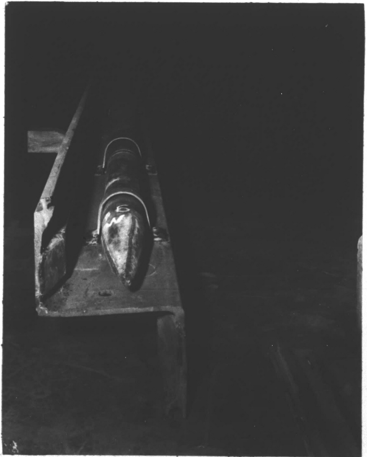
Fig. 9 - Channels Over SR4 Gages and Slope Indicator Pipe at Bottom of Instrumented Sheet Piling
